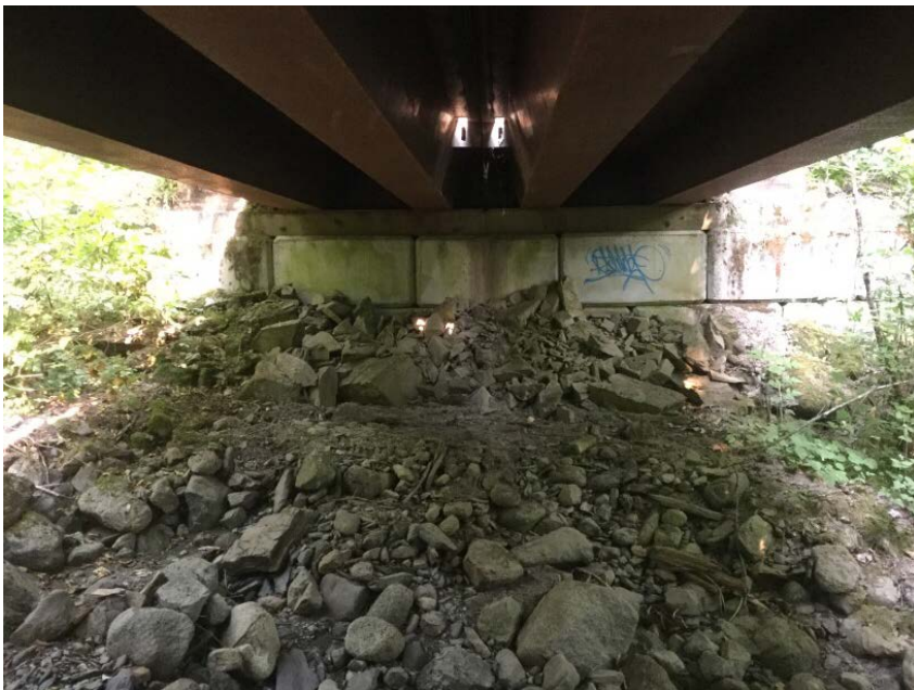
Left Bank Abutment when facing downstream
