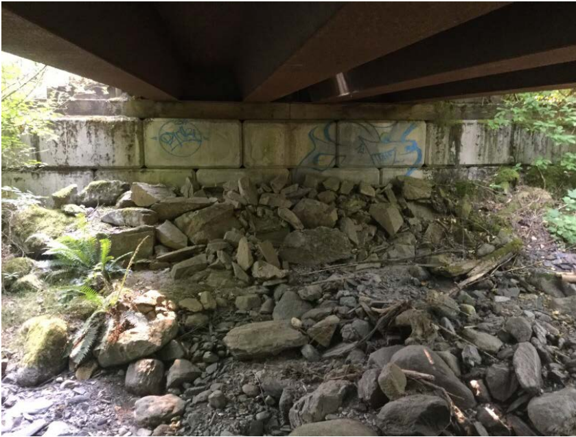
Right Bank Abutment when facing downstream
