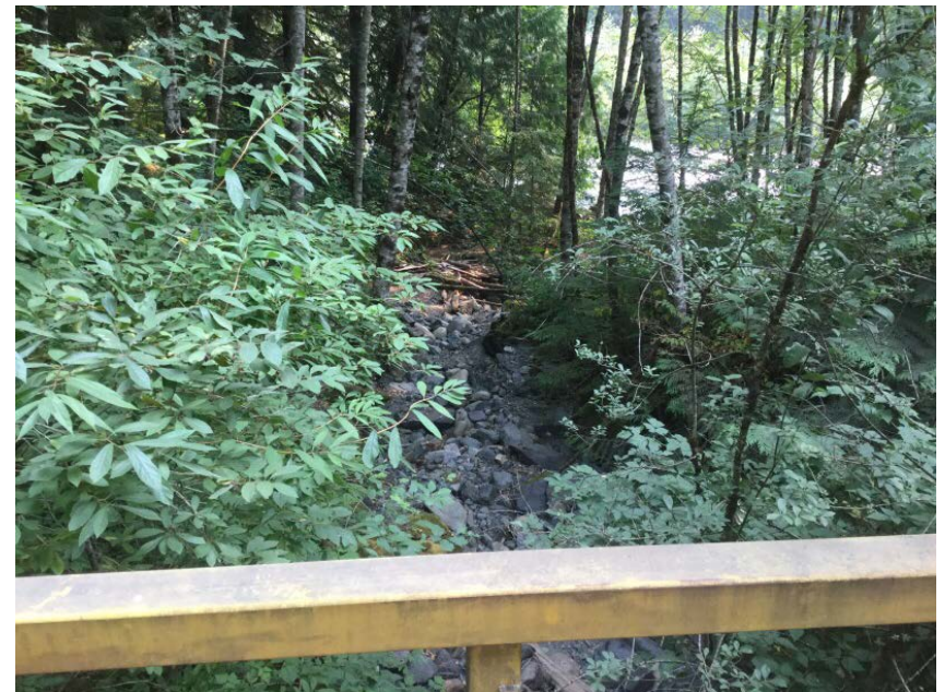
Looking downstream from deck
